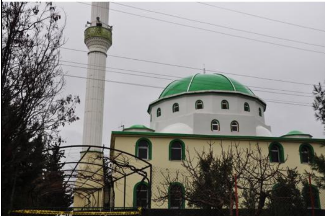
Figure 4. Damage cost is nearly zero in Cigdemtepe (Crocushill) which is adjacent to the epicenter
