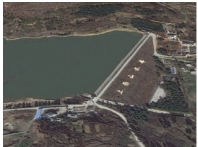
Figure 2. Actual view of the project
