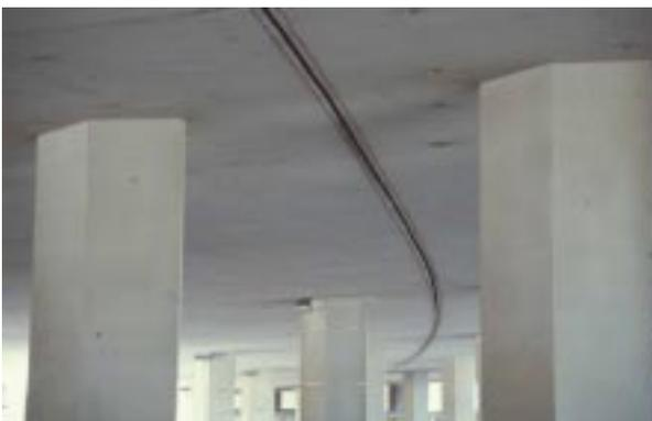
Fig. 3 "Diamond" columns and the longitudinal hinge of the viaduct
