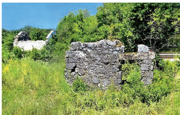
1941. - 1943. - ostaci ruševine preko ceste naše kuće u kojim je boravila talijanska vojska za osiguranje pruge Zagreb – Split 1941 - 1943 - Remains of ruins across the street from our house where the Italian army stayed to secure the Zagreb - Split railway.
