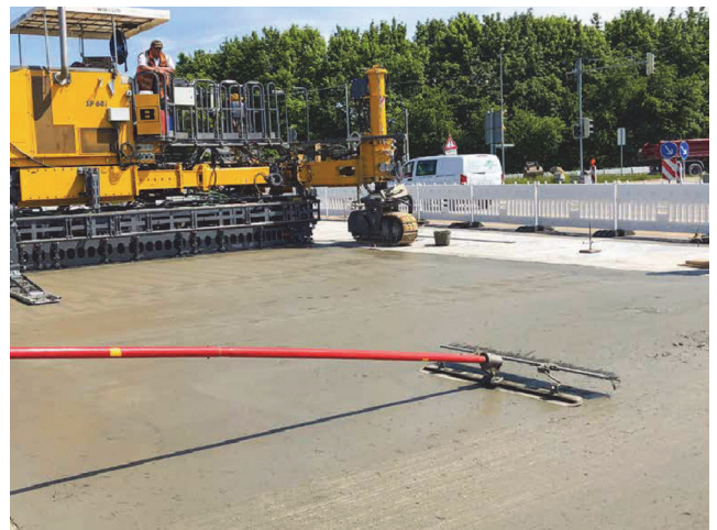
Figure 13. Application of broom finish [3]
