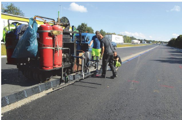
Figure 22. Precise bonding of bituminous sheets to asphalt cut edges [7]
