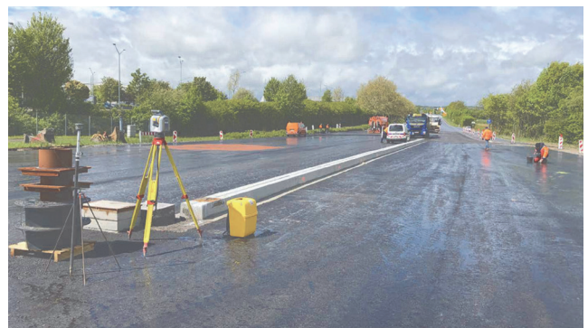
Figure 6. Concrete construction junction: asphalt base-course, Daimler junction [3]
