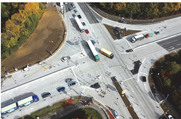
Figure 3. Concrete construction junction: Daimler Junction, Boeblingen District [3]
