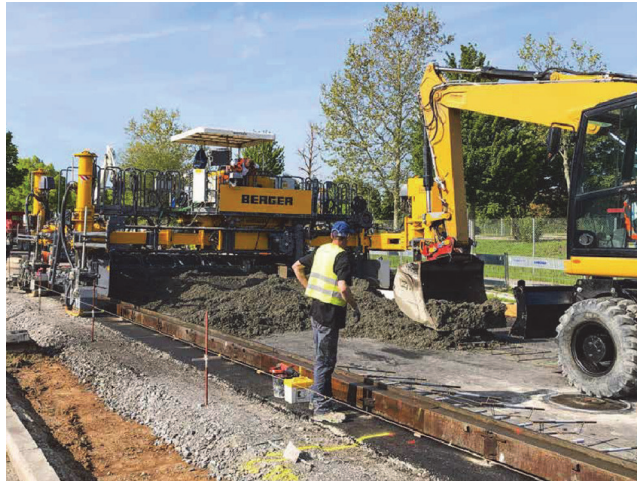
Figure 12. Initial "start-up" during the road paver production [3]
