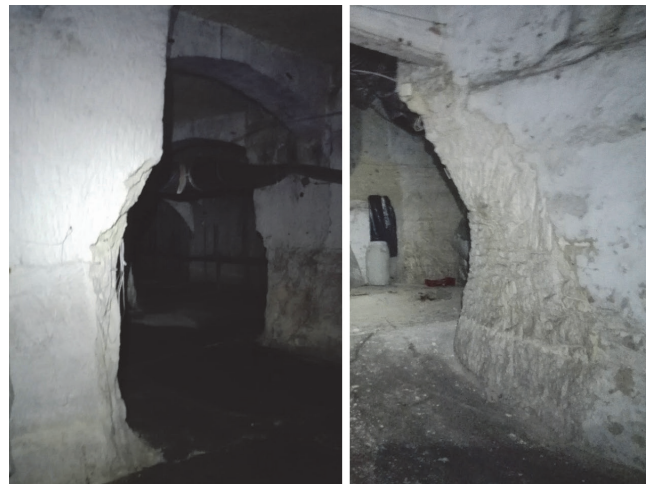
Figure 1. The cut pillars in the studied area
