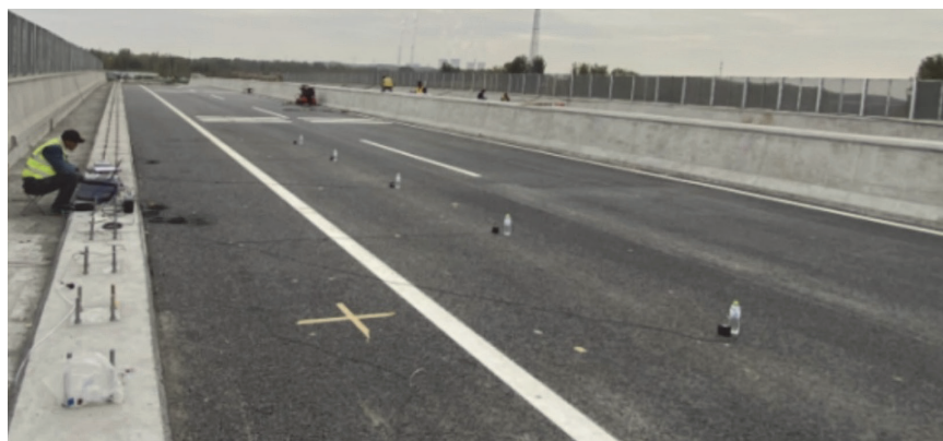
Figure 10. Field photograph of the modal test
