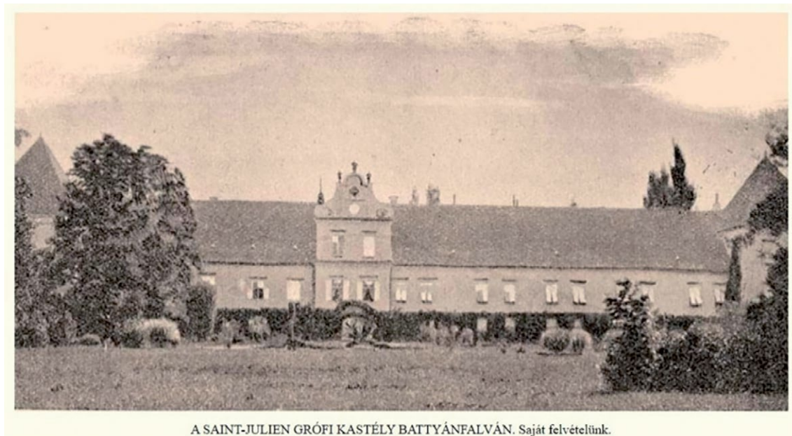
Fig. 11 This photograph was taken in 1898 at the west side of the manor house, from the adjacent park, showing the more representative entrance with a avant-corpes . The ivy covering the lower level of the mansion is also evident. According to the inscription on the photograph, Saját felvételünk ('personal photograph'), it was taken by Borovszky Samu (1860-1912), a Hungarian historian who became a member of the governing board of the Historical Society in 1889 and a corresponding member of the Academy since 1899 (source: https://www.arcanum.com/hu/online-kiadvanyok/Borovszky-borovszky-samu-magyarorszag-varmegyei-es-varosai-1/vas-varmegye-1C4AE/vasvarmegye-kozsegei-1C5BD/battyanfalfa-saint-julien-kastely-1C629/ (4. 12. 2023)).
