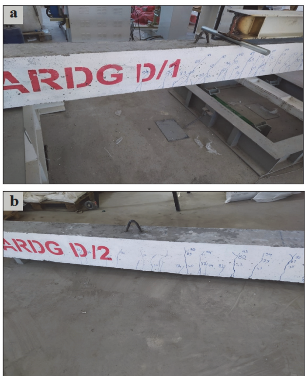
Figure 5 Flexural and shear cracks of straight post-tensioned beam (a) POSTTENST/1, (b) POSTTENST/2
