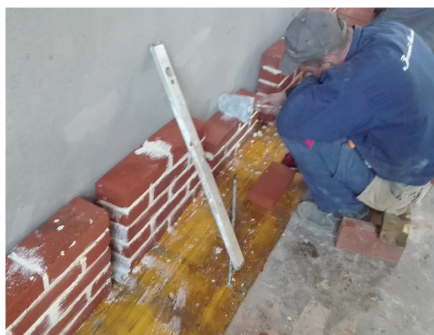
Figure 6. Construction of test specimens
