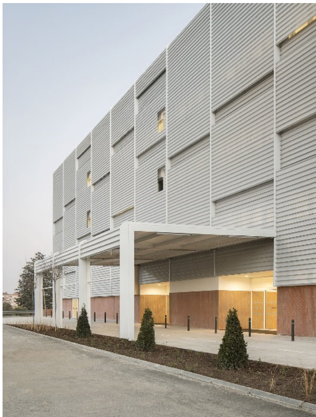
Fig. 7: Photograph of hospital project in Lérida applying BIM. BIM, building information modelling.
