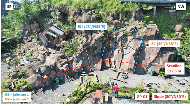
Figure 11: Kinematic analysis results and drone photo of section GP-01
