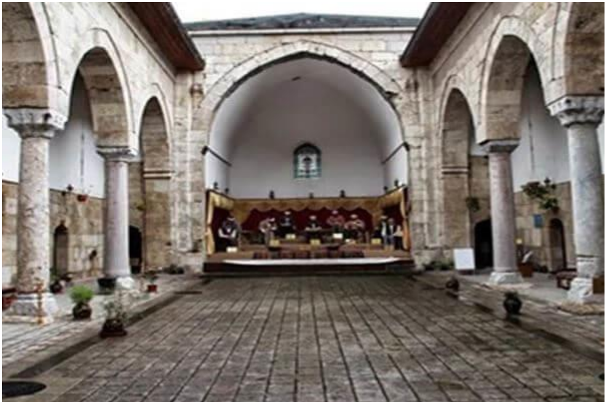
Figure 3A/B. Amasya Darüüşşifa (Central State University Hospital), est. 1308. External/Internal (A/B) view respectively.
