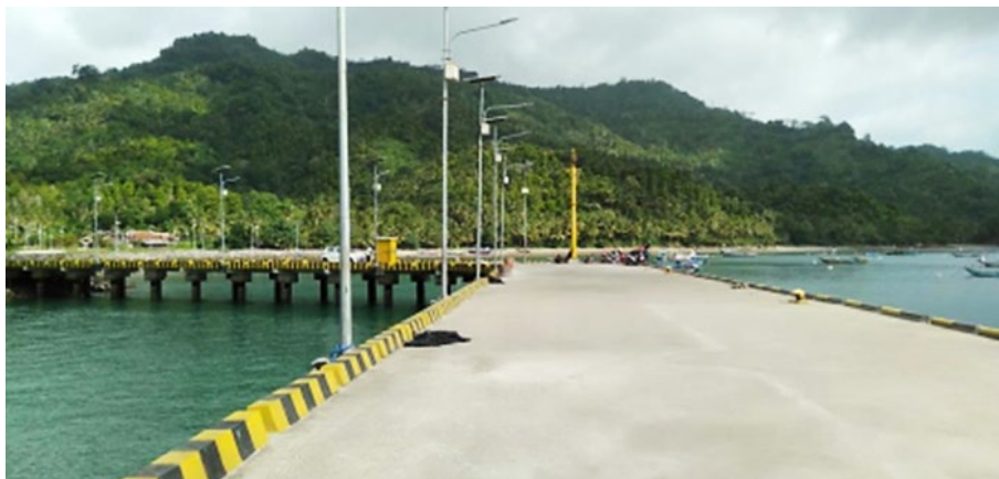
Figure 11. Prigi Commercial Port Pier in Watulimo District, Trenggalek Regency
