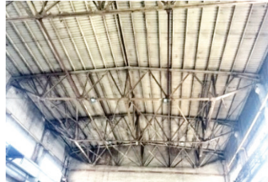
General view of the trusses
