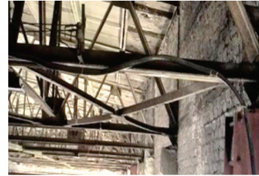
Curvature of the truss's elements
