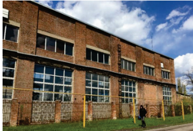
General view of industrial building
