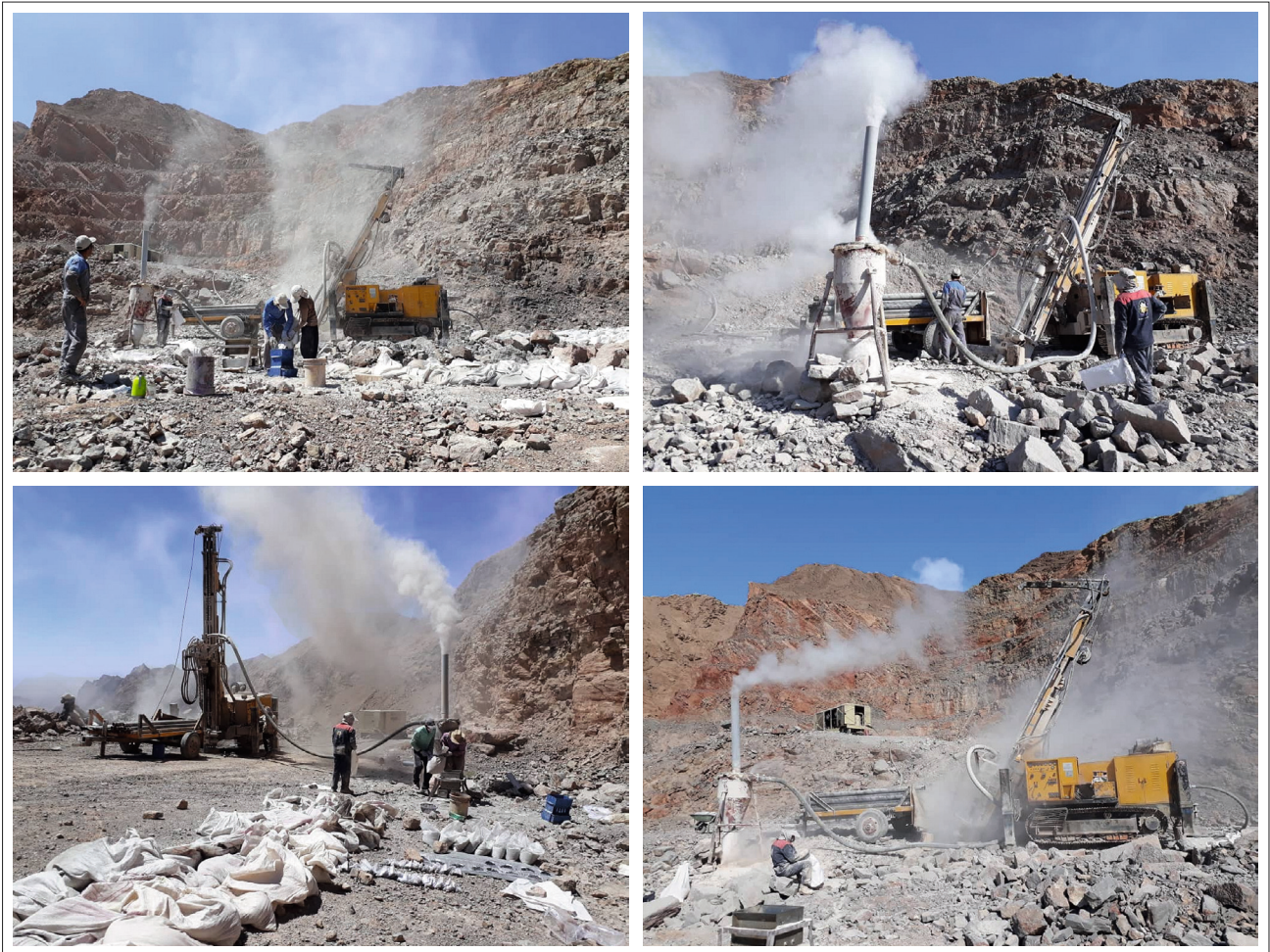
Figure 4: Views of excavation and sampling activities related to exploration boreholes identified using DGPR results at the Yazd calamine mine.
