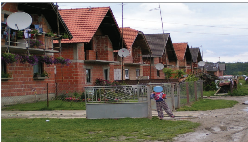
Fig. 23 Newer construction of a Roma settlement, buildings without façades
