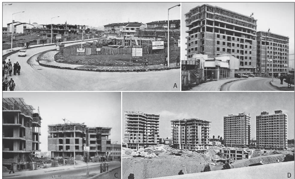
FIG. 6 ADVERTISEMENTS IN THE MİLLİYET NEWSPAPER FIG. 7 PHOTOGRAPHS FROM THE ABIDE SITESİ CONSTRUCTION: (A) 1976, (B) 1977, (C) 1976, (D) 1977
