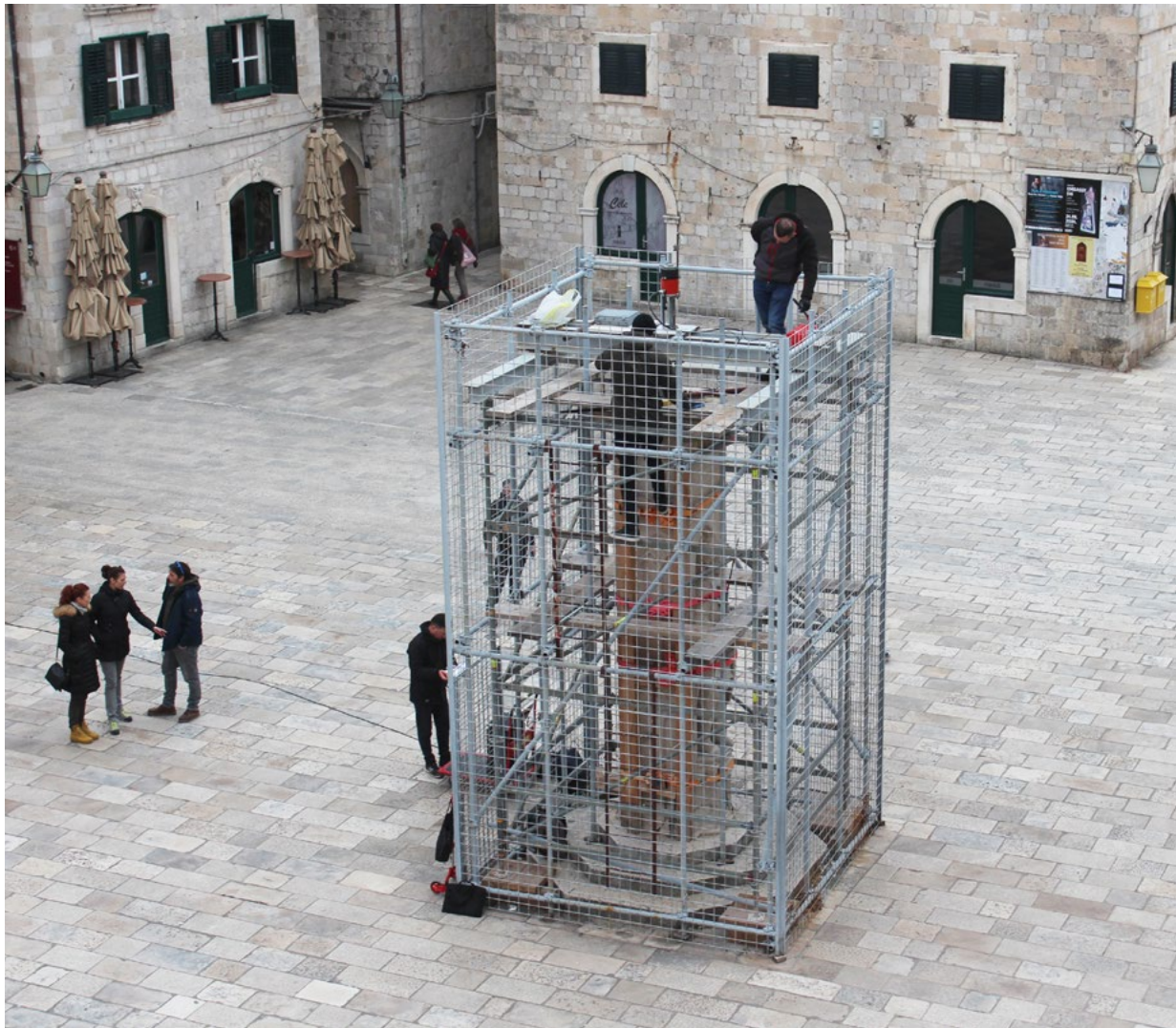
16. Orlando's Column, pokušaj otpuštanja sile na centralnom trnu uz pomoć hidrauličke preše (arhiva GDU, 2024.) Orlando's Column, an attempt to release the force on the central mandrel with the help of a hydraulic press (GDU archive, 2024)
