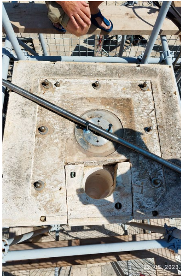
14. Orlandov stup, pokušaj ručnog popuštanja sile centralnog stupa (arhiva HRZ-a, snimka: V. Marinković, 2023.) Orlando's Column, an attempt to manually release the force on the central pillar (HRZ Archive, V. Marinković, 2023)
