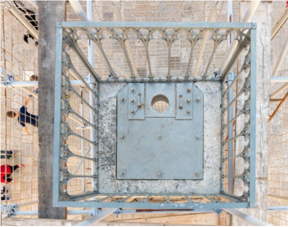
7. Orlando's Column, view from above, stainless steel cover (HRZ Archive, P. Gamulin, 2021)
