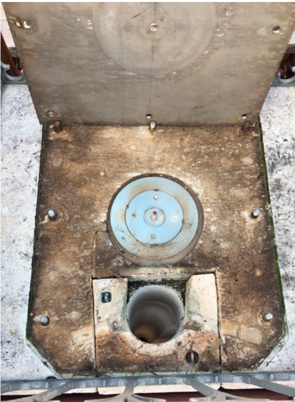
8. Orlando's Column, view from above, central thorn with nut (HRZ Archive, V. Marinković, 2020)
