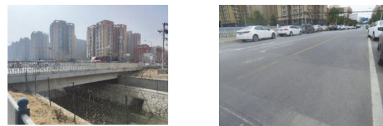
Figure 6 Youyi Drain Crossing Bridge
