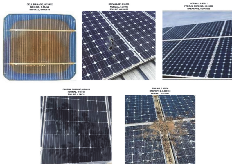
Figure 7 Testing results of PV fault classification
