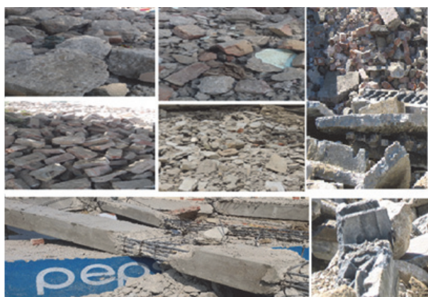
Figure 1 Demolished wastes of structural elements
