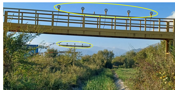
Figure 6 Compact portal over the stream with crossbar of the Tivat Airport approach lighting with maintenance platform, [13]
