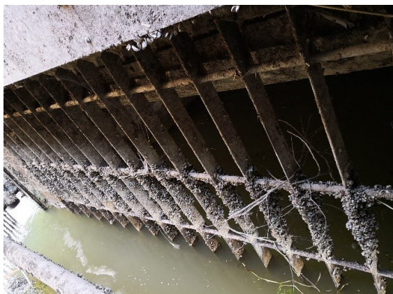
Slika 5. Gruba rešetka agC HE Dubrava Figure 5. Rough grid agC HPP Dubrava
