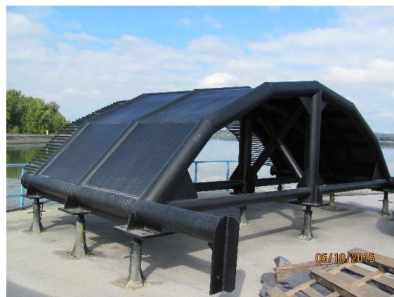
Slika 7. Obnova antikorozivne zaštite Figure 7. Restoration of anti-corrosion protection
