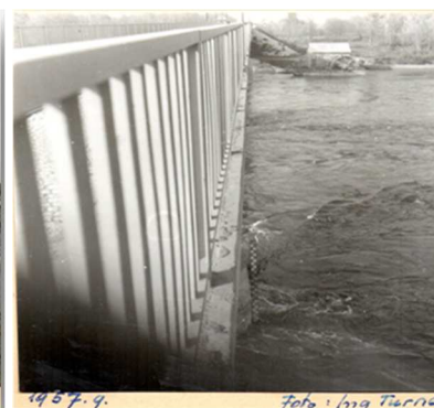
Figure 3 Water gauge on the bridge pillar on the downstream side Photo: Turner, 1957 (DHMZ)
