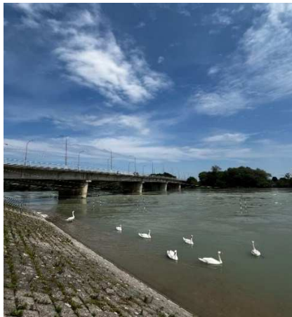
Figure 7 New road-rail bridge Varaždin – Čakovec, June 24, 2024, Photo: Maloić, J.
