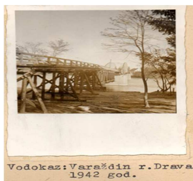
Figure 1 Damaged bridge in 1942, water gauge relocated to the right bank (DHMZ)
