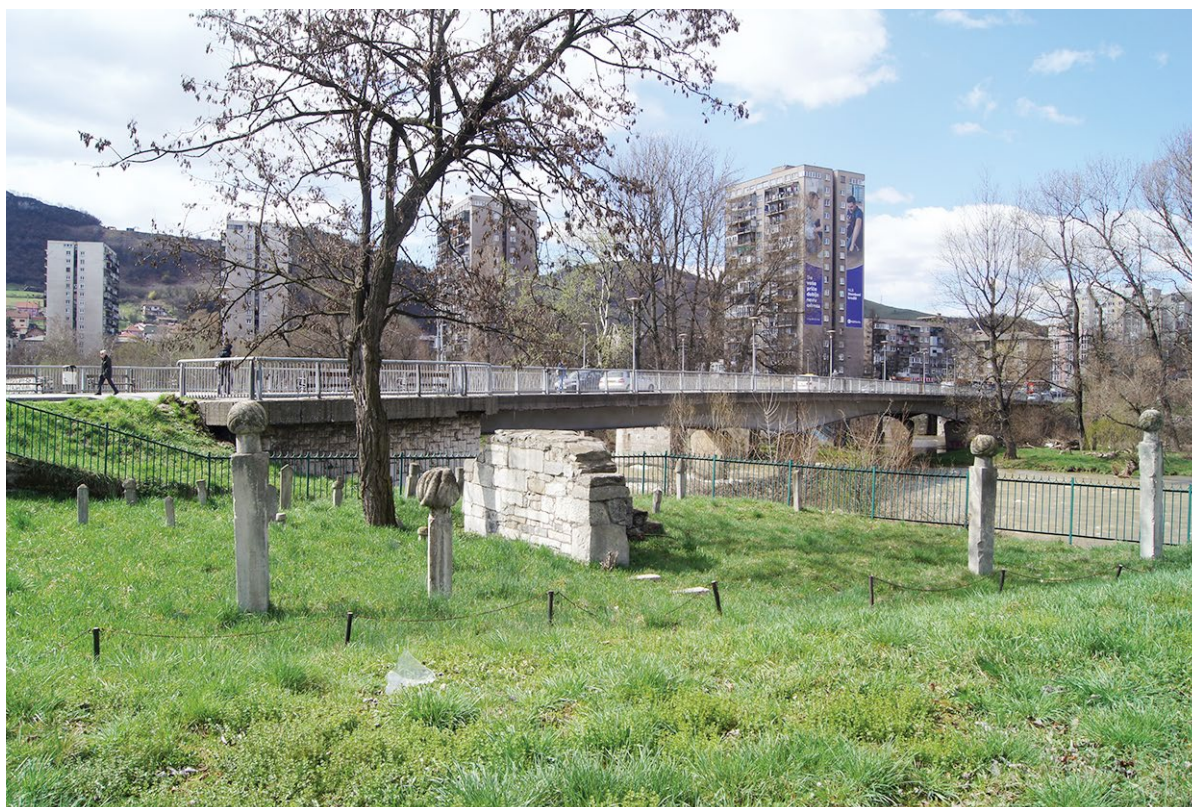
FIGURE 8 The new bridge built in 1969
