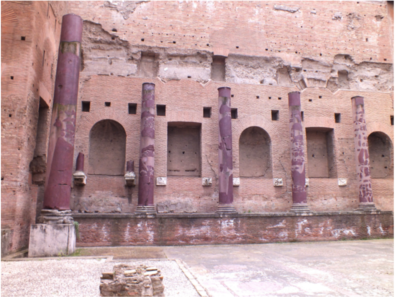
Figure 4. Rome, Temple of Venus and Rome. Porphyry shafts inside the cells: flanking the apses, on the side walls and in the internal niches (photo: J. Á. Domingo).
