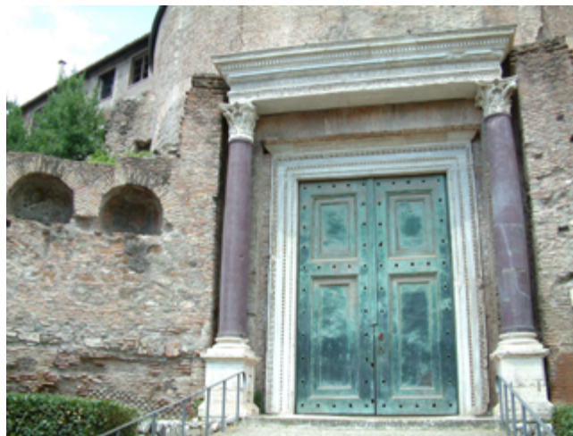
Figure 3. Rome, Temple of Romulus. Porphyry shafts flanking the entrance (photo: J. Á. Domingo).
