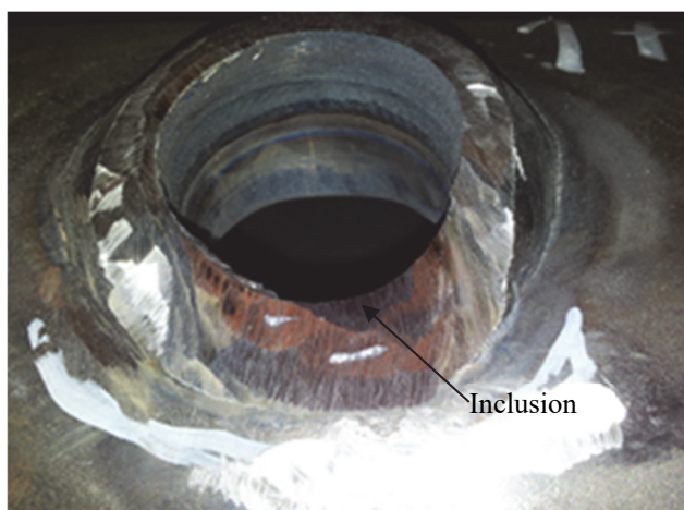
Figure 1 Grinded macro-sample of welded joint with inclusion
