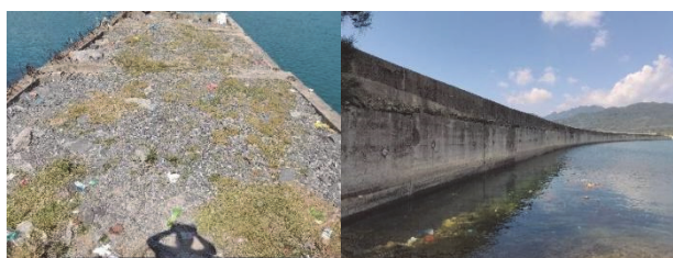
Figure 15 Along Wanning Sun Island (a) Tank along Wanning Sun Island; (b) Vertical retaining wall along Wanning Sun Island
