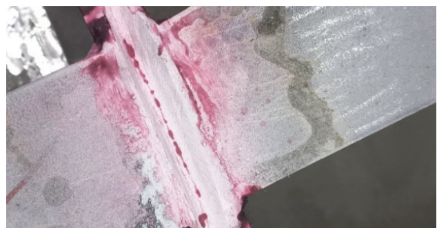
Figure 21 PT examination of welded joint no. 1 after repair
