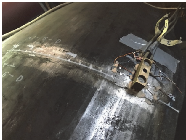
Figure 6 Residual stress measuring position on vessel head
