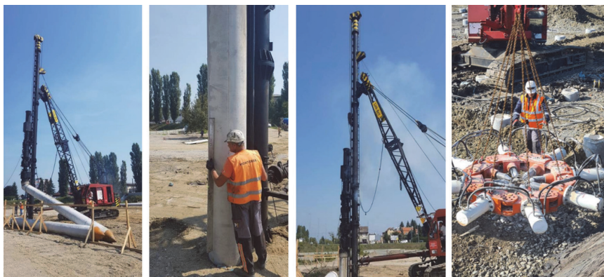
Figure 1. Technology of implementation of driven piles (lifting, positioning, driving, preparing the pile head with pliers)
