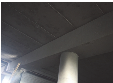
Figure 5 Bridge upper structure
