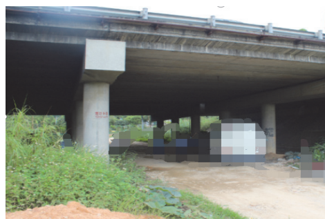
Figure 3 Bridge facade illumination
