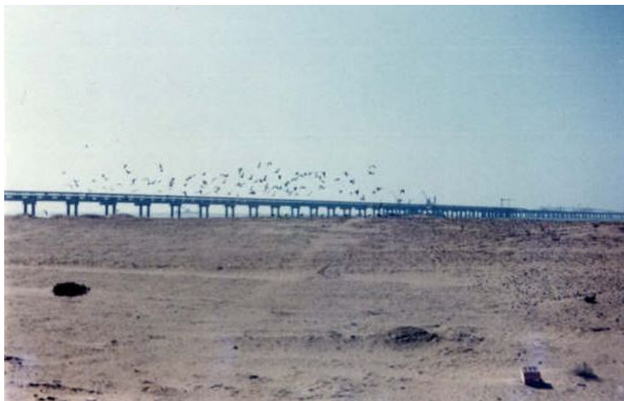
Slika 5. Najduži trakasti transporter na svijetu, dug 100 km, u Zapadnoj Sahari Figure 5. The longest belt conveyor in the world, 100 km long, in Western Sahara
