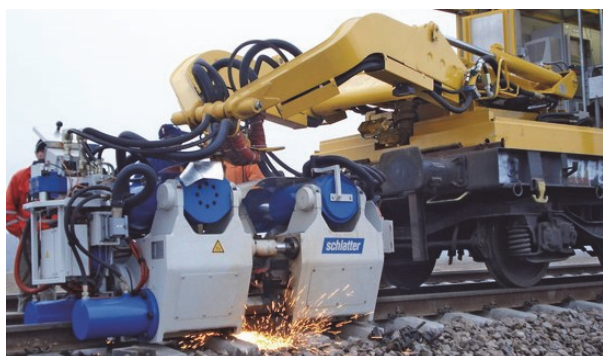
Figure 5 Mobile flash butt welding machine
