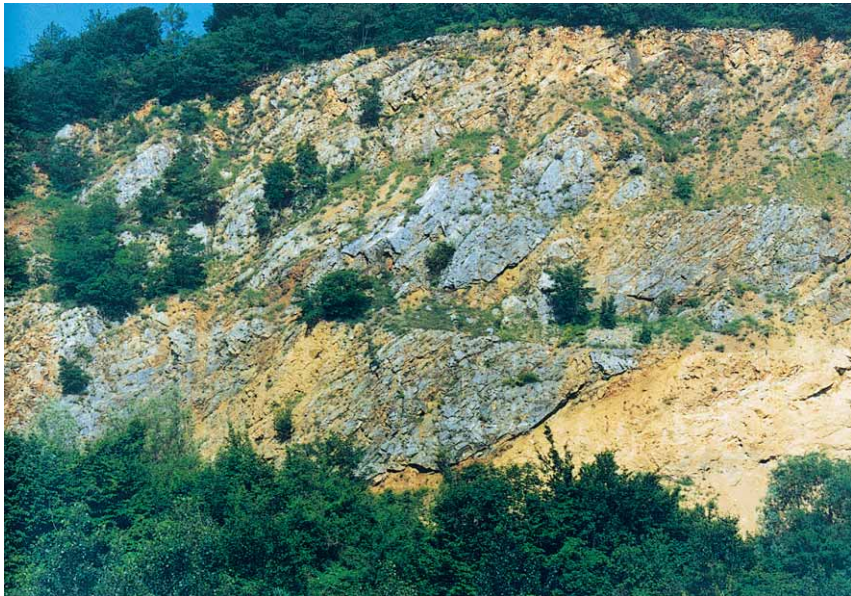
Fig. 21. Markuševac quarry. Reverse faults and R_1 fracture system in the slightly metamorphosed limestones of the Markuševac member.
