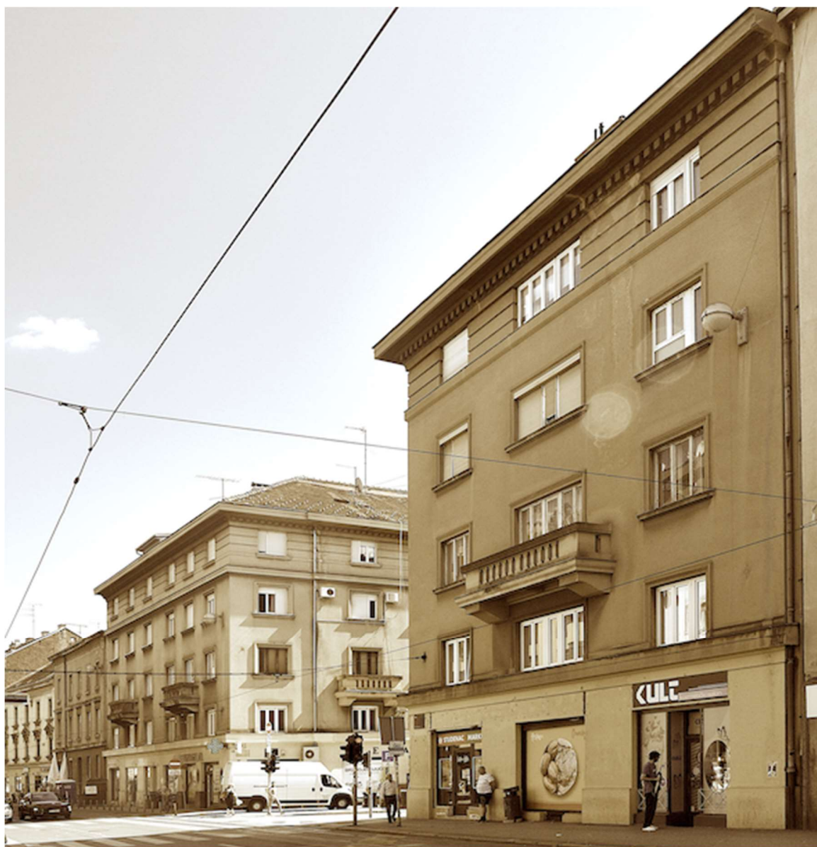
Figure 2. Construction company Monjac, Krušlin and Behrmann: corner building Monjac – Krušlin at Ilica 139 A / Slovenska Street 1 and at Slovenska Street 2 from 1930.
