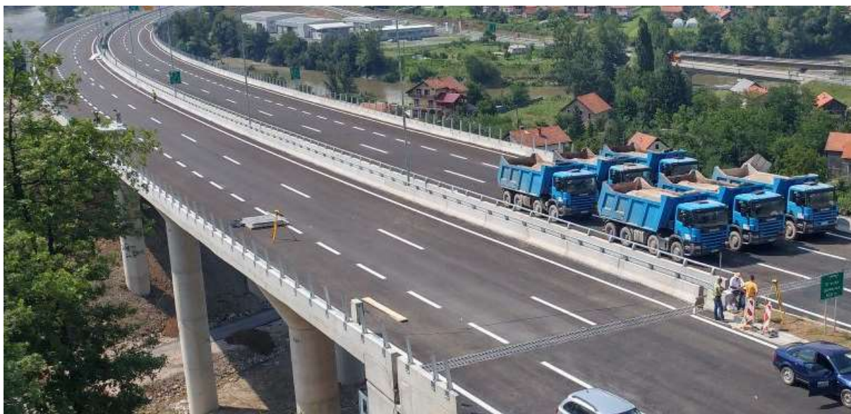
Figure 8. – Load placed in position
