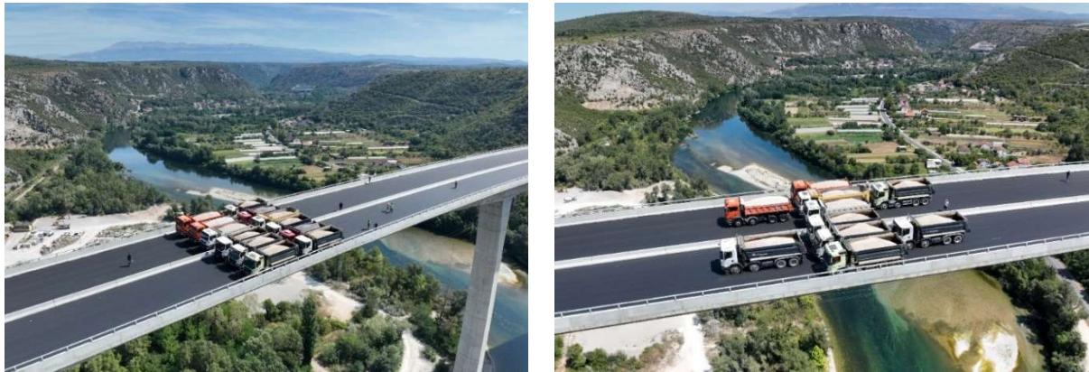
Figure 12. - Placing the load in position for static testing
