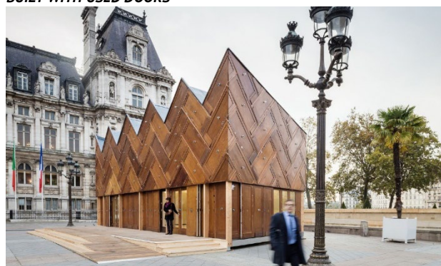
FIGURE 1. ANALITICAL APPROACH TO UPCYCLING AS AN ARCHITECTURAL MANIFESTO. LE PAVILLON CIRCULAIRE IN PARIS BUILT WITH USED DOORS
