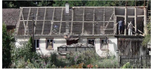
FIGURE 4. HISTORICAL BUILDING BEFORE RETROFITTING
