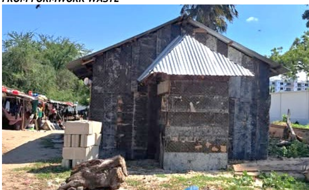
FIGURE 2. ORGANIC APPROACH TO UPCYCLING AS AN EVERYDAY ARCHITECTURAL REALITY. A BUILDING IN DAR-ES-SALAAM BUILT FROM FORMWORK WASTE
