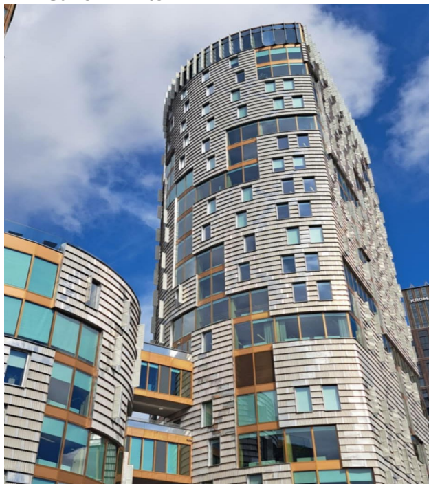
FIGURE 3. ANALITICAL APPROACH TO UPCYCLING AS A TOOL OF THE CIRCULAR ECONOMY. A BUILDING BUILT FROM USED LETTERBOXES IN AARHUS
