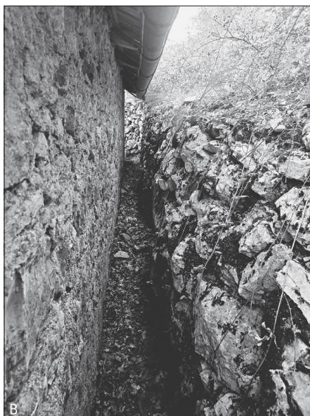
FIG. 5 A) RETAINING WALL EMBEDDED IN THE GROUND – NOŽNJE; B) SPECIFIC WALL SOLUTION WHERE THE COMPACTED SOIL LAYER IS MISSING – POD GREDA
