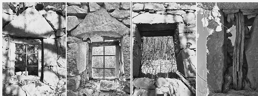
External and internal view – Pod
