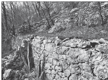
FIG. 5 A) RETAINING WALL EMBEDDED IN THE GROUND – NOŽNJE; B) SPECIFIC WALL SOLUTION WHERE THE COMPACTED SOIL LAYER IS MISSING – POD GREDA
