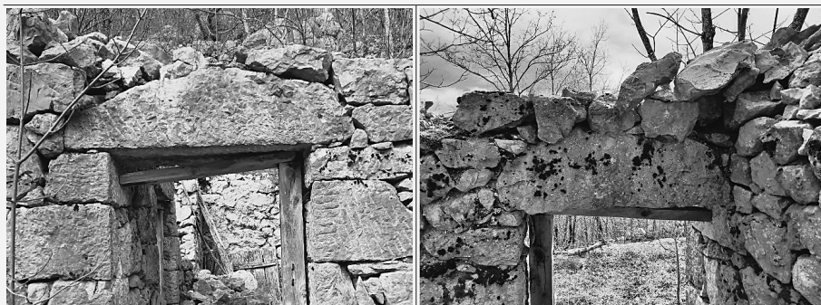
External and internal view – Noznje
