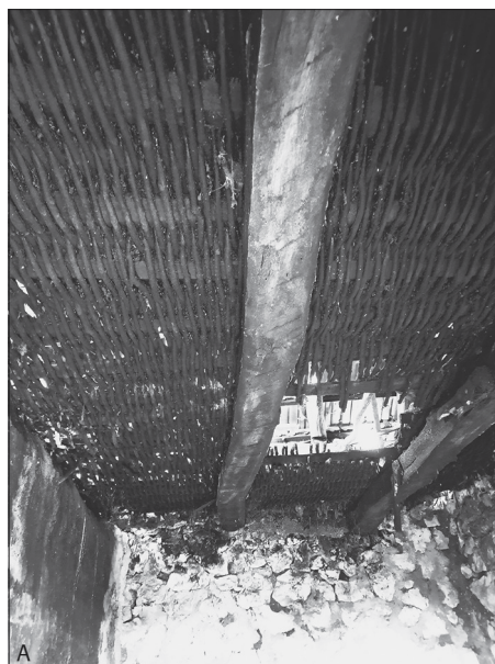
FIG. 8 ILLUSTRATION OF TWO TYPES OF CEILING: A) BEAMS AND WOVEN BRANCHES – LISA; B) BEAMS AND PLANKS ARRANGEMENT – TRENICA
