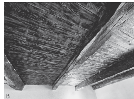
FIG. 8 ILLUSTRATION OF TWO TYPES OF CEILING: A) BEAMS AND WOVEN BRANCHES – LISA; B) BEAMS AND PLANKS ARRANGEMENT – TRENICA
