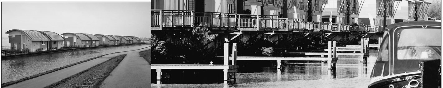
FIG. 6 AMPHIBIOUS HOUSING IN MAASBOMMEL, NETHERLANDS – RESIDENTIAL UNITS RESTING ON THE GROUND UNDER NORMAL CONDITIONS AND FLOATING DURING FLOODS VIA CONCRETE PONTOONS. THE PROJECT DEMONSTRATES A LOW-TECH YET SCALABLE MODEL FOR CLIMATE ADAPTATION IN FLOOD-PRONE AREAS.
