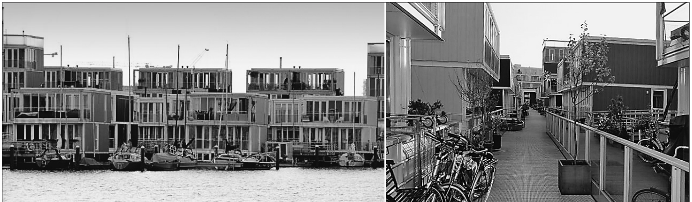
FIG. 2 VIEW OF WATERBUURT-WEST FLOATING NEIGHBORHOOD, IJBURG, AMSTERDAM
