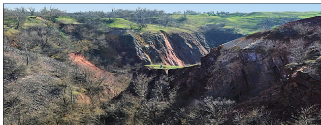
Figure 11. Sinkhole No. 2 (photo by Dmitry Antonov, 2015)
