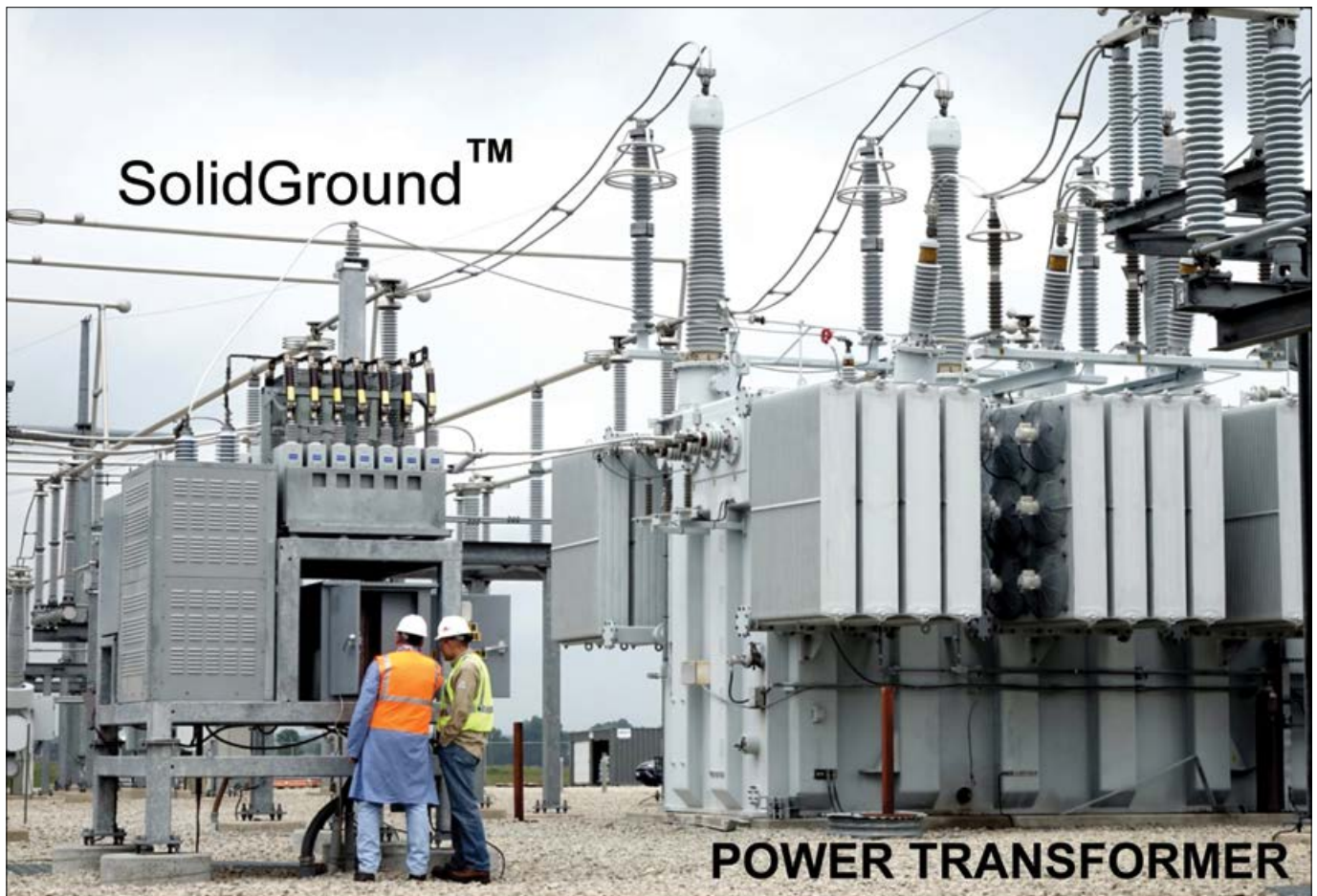
Figure 3. SolidGround™ [4] by ABB (left) is meant for blocking GIC in a neutral conductor of a power transformer (right)
