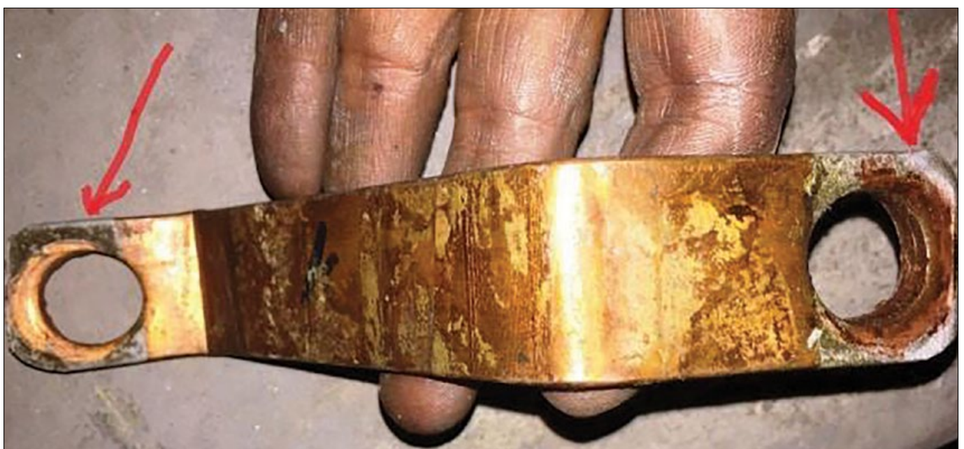
Figure 9. Severe oxidation on the core-ground connection, resulting in poor contact by [7].
