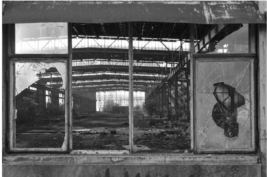
Picture 8. Remnants of construction machinery "Radoje Dakić" plant in Podgorica, photo: I. Laković.
