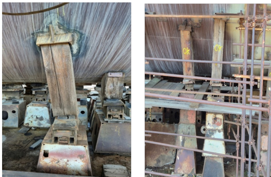
Figure 2. Condition of slipway equipment [1]
