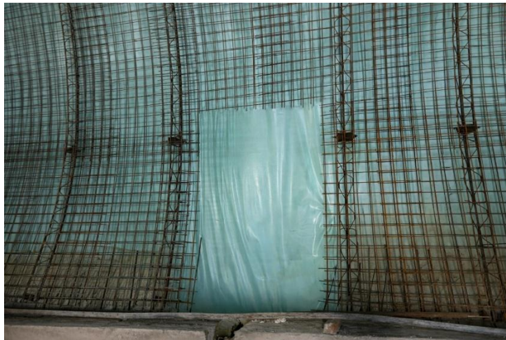
Figure 7. Waterproofing within the inspection niche, Kobilja Glava Tunnel [5]
