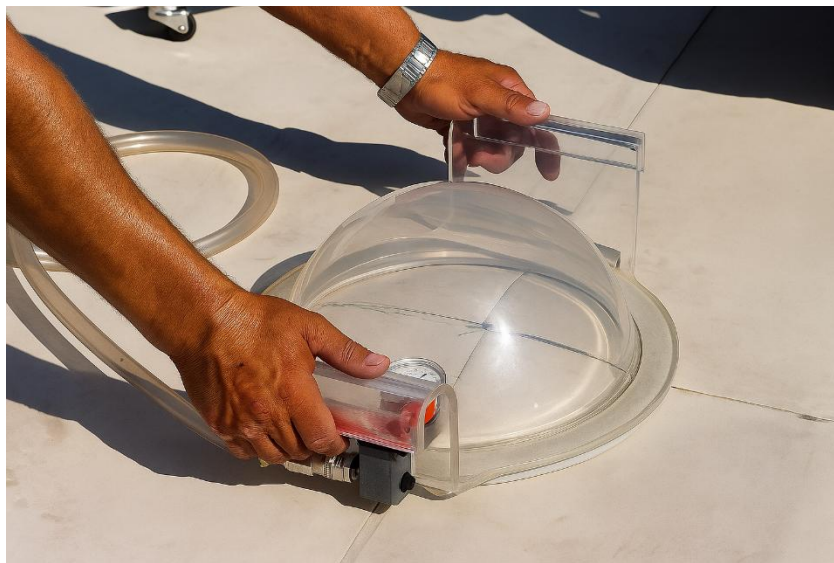
Figure 9. Testing of the membrane using the vacuum method [1]
