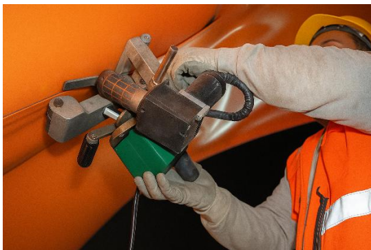
Figure 4. Illustration of a double weld [4]
