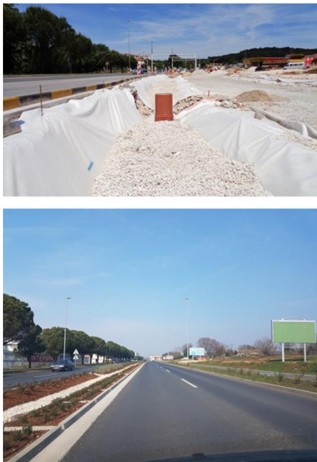
Figure 6. City bypass under construction and after planting (Starum) [10]
