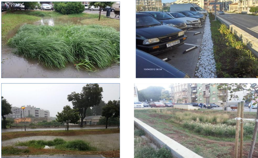
Figure 5. Constructed NbS on Nazorova Street (Starum) [6]
