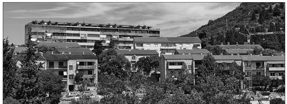
FIG. 8 RESIDENTIAL BUILDING, THE SO-CALLED BLOK (ARCH. IVO GERSIĆ) ABOVE RESIDENTIAL BLDGS. IN ROGOTINSKA AND VLADIMIRA NAZORA STREETS, SOURCE: DUJE JELČIĆ
