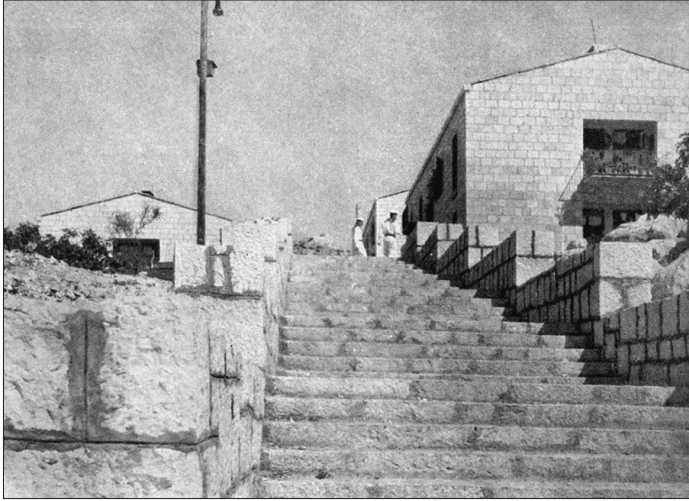
FIG. 5. PHOTOGRAPH OF RESIDENTIAL BUILDINGS AT PRISNICA (ARCH. LOVRO PERKOVIC), SOURCE: ***(1955)
